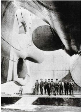
Do you see the propeller? There were three of them. As the giant engines turned them with 50,000 horsepower, the humongous ship was pushed forward at about 23 mph. Now they are at the bottom of
