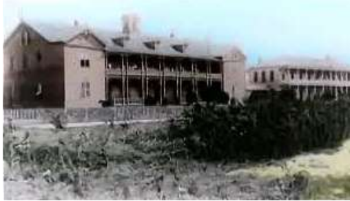
Just off the sand of the beach is St. Mary's orphanage.
